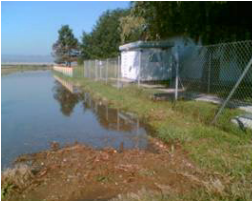
Slika 1. Stanje na avtomatski merilni postaji Levec Spodnja Savinjska dolina tri dni po neurju Figure 1. Situation at automatic measuring station Levec Lower Savinja valley three days after storm
